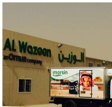
Completion of cheese manufacturing facility in Riyadh, Saudi Arabia
